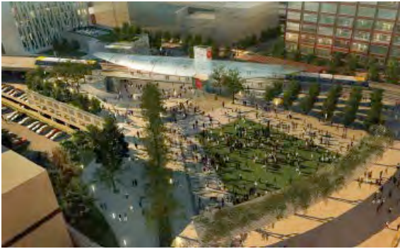
Target Field Station Minneapolis, Minnesota
