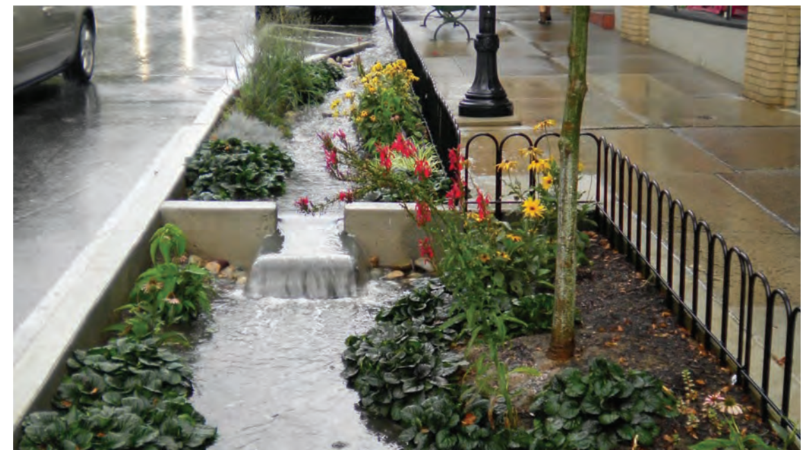
Stormwater flowing through a system that is similar to, but a smaller scale than the proposed tree trench
