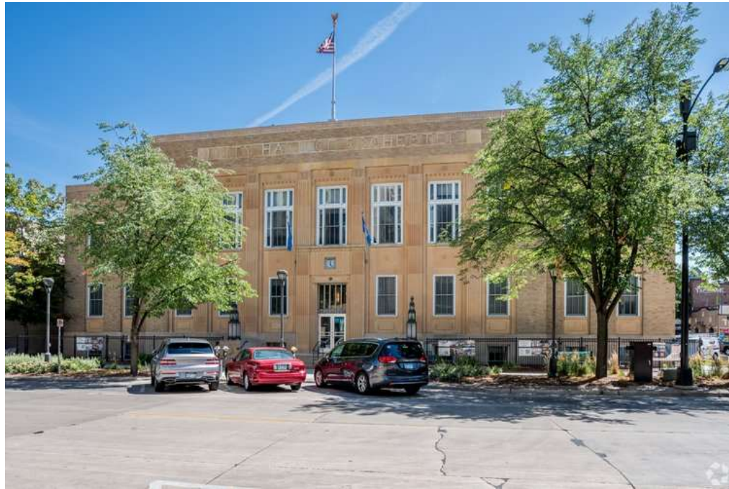
224 First Ave SW
