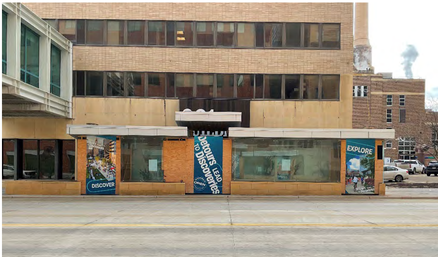
Wayfinding installation on 2 nd Street SW bus terminal.
